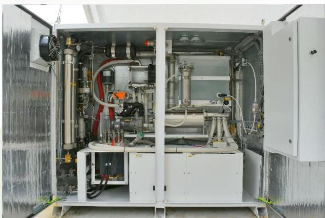
Photograph of the 60kW PEM electrolyzer used in the first U.S. pilot of P2G
