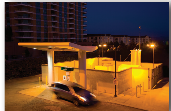
Figure 1. GEN III Hydrogen Refueling Station at Night (Photo Credit: Paul Kennedy)
